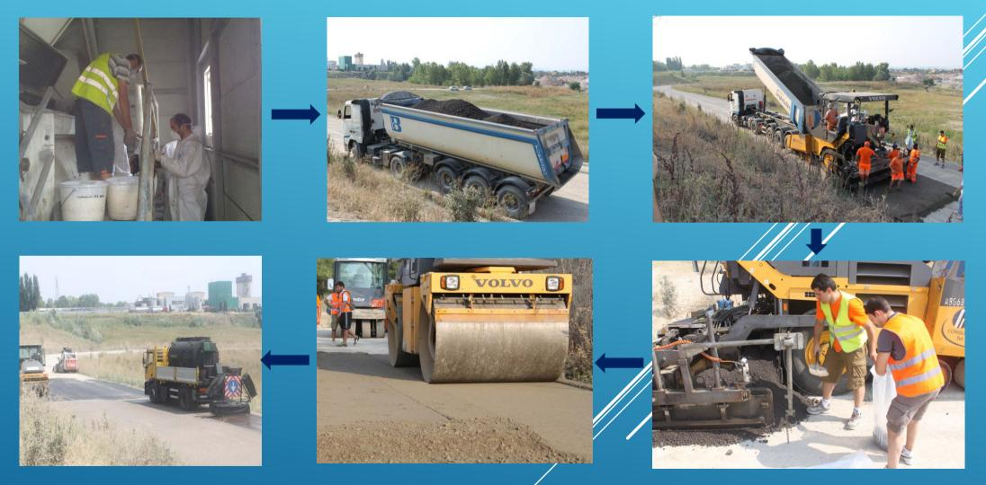
During paving, loose samples were collected at the paver screed and immediately compacted with the gyratory compactor available in the quarry laboratory.
